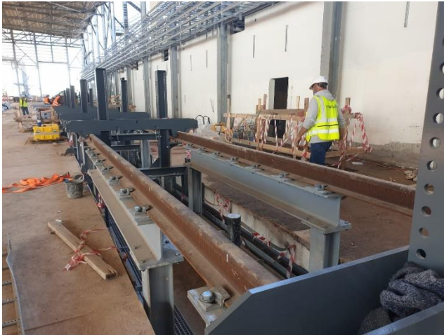
Assembly and levelling of the tracks
