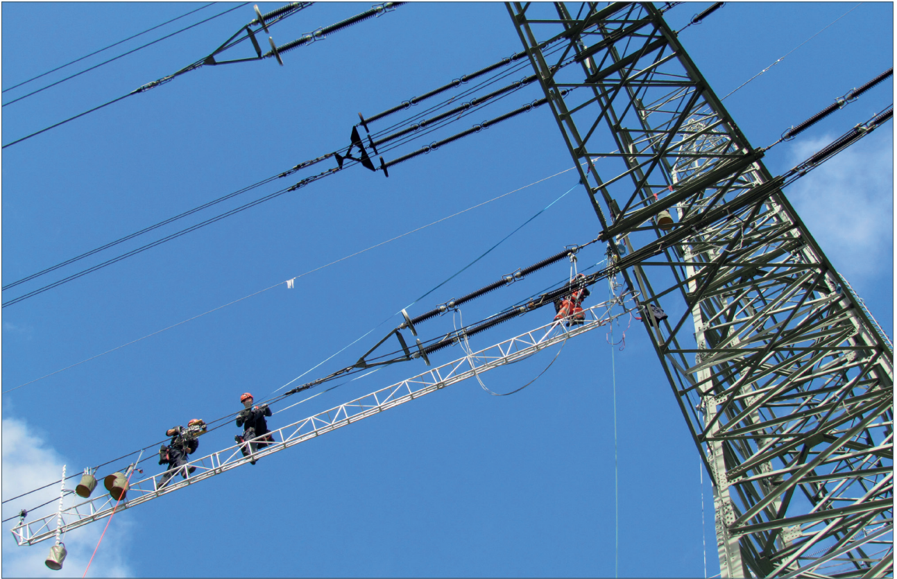
Overhead line construction
