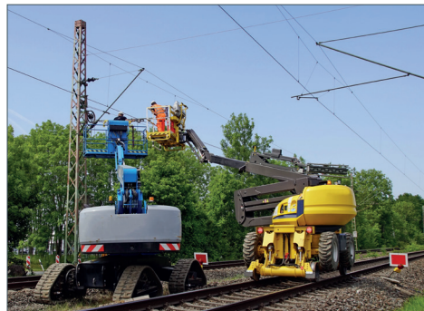
Construction of contact lines
