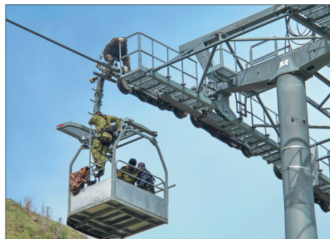
Cable car construction
